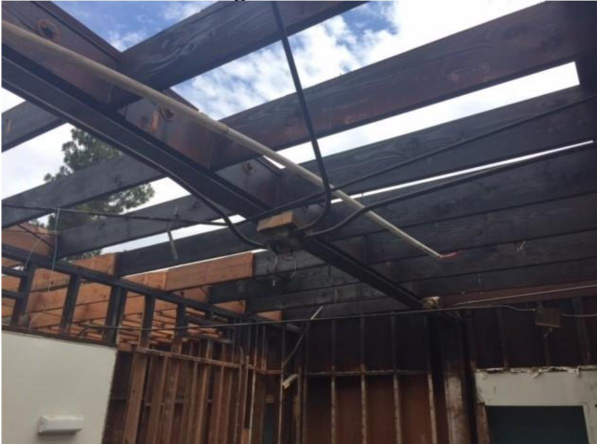
Old fire damage discovered during construction
