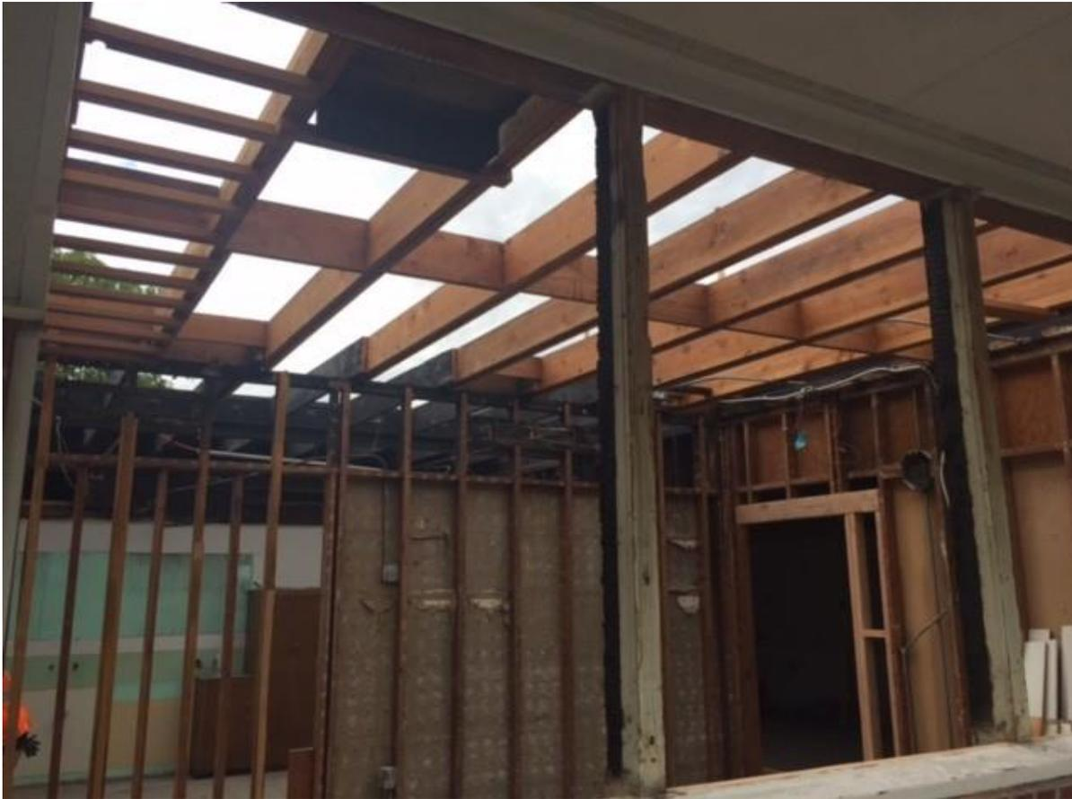
Administration office stripped to studs, roofing replacement due to discovery of fire damage
