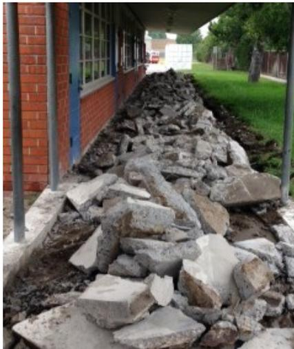
*Demolition of concrete required for path of travel*
