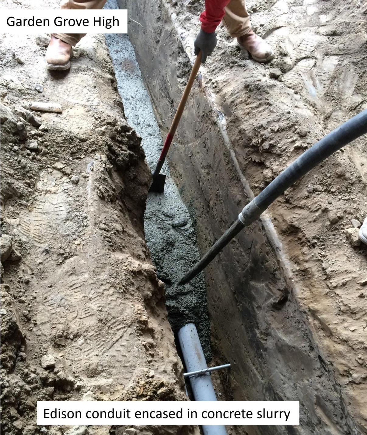
Edison conduit encased in concrete slurry
