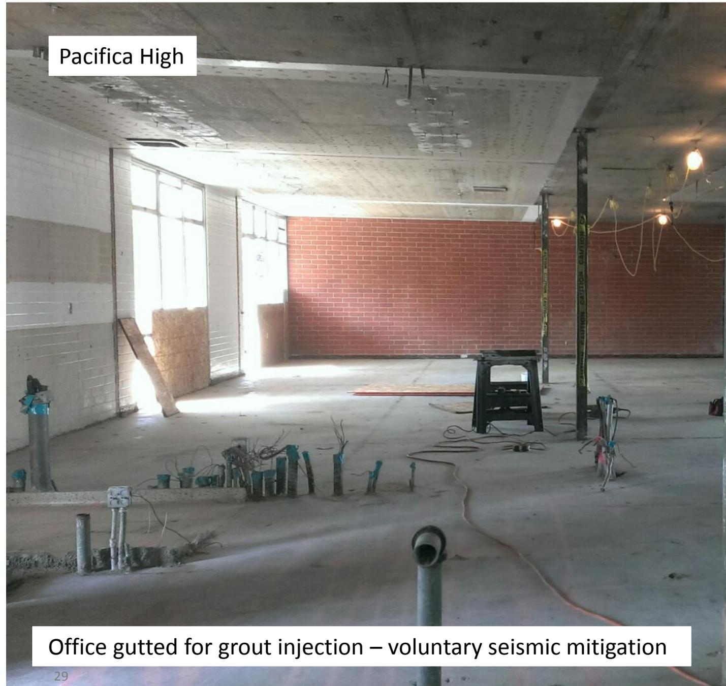
Office gutted for grout injection – voluntary seismic mitigation
