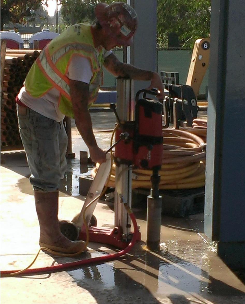
Core drilling for grout injection
